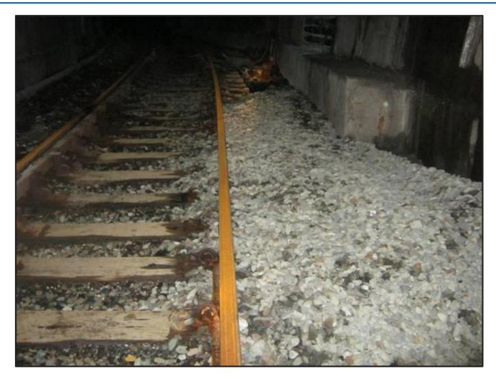
Corroded rail and fouled ballast in Tunnel F (11/3/2012)
